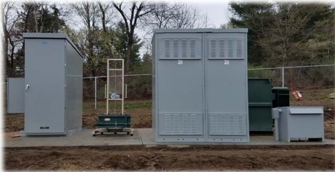
Figure 1: Medium Voltage Utility Intertie Switchgear, Step-Up Transformer, Low Voltage Combiner Switchboard, & Grounding System Outdoor Pad mount NEMA 3R Non-Walk-In
