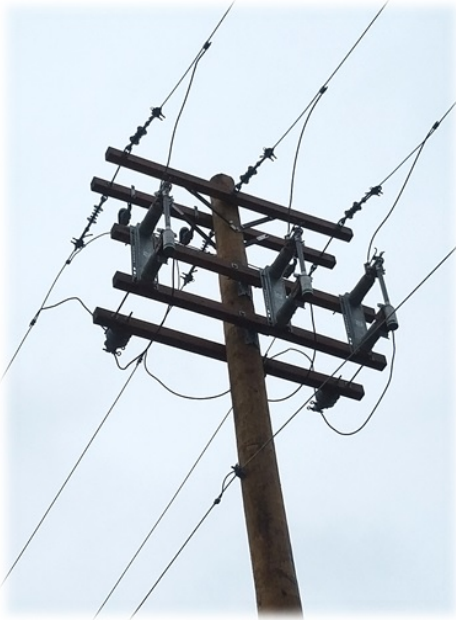
Figure 2: Pole Mount Fused Cutouts Disconnect Switches
