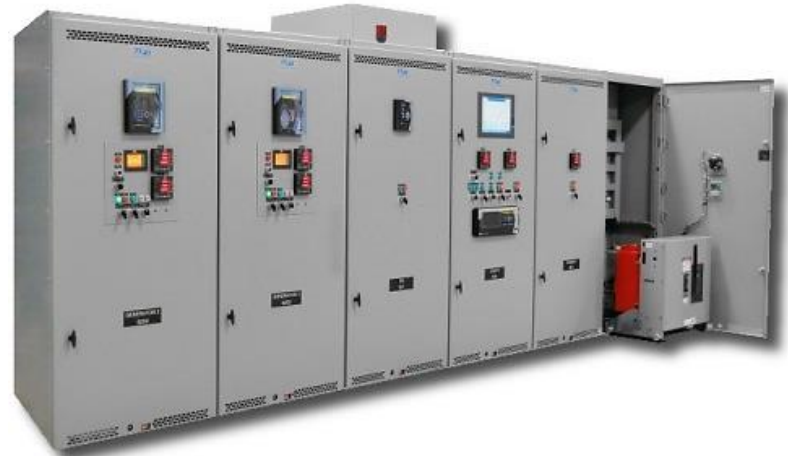
Figure 1: Medium Voltage Multiple Genset Utility Paralleling Lineup
