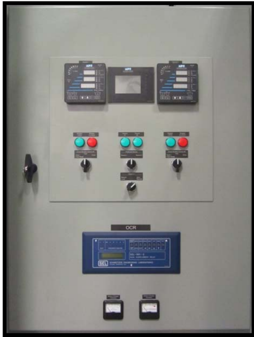
Figure 4: Standard Automatic Transfer Control Panel
