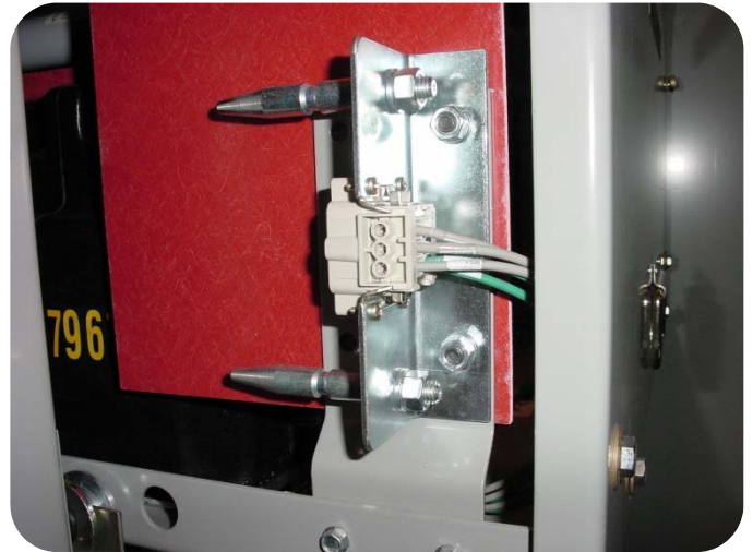
Figure 12: Self-Aligning Drawer Contacts
