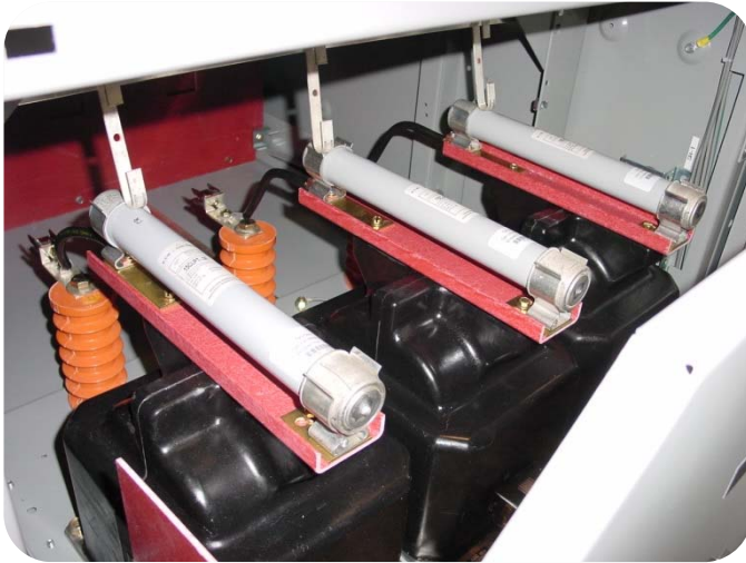
Figure 11: Inside Voltage Transformer Drawer
