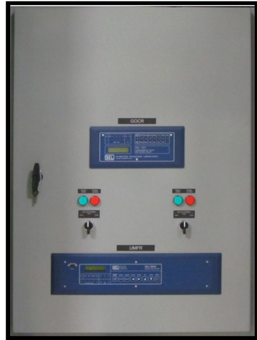
Figure 5: Optional Basic Circuit Breaker Control Panel with Automatic Transfer Control by Others
