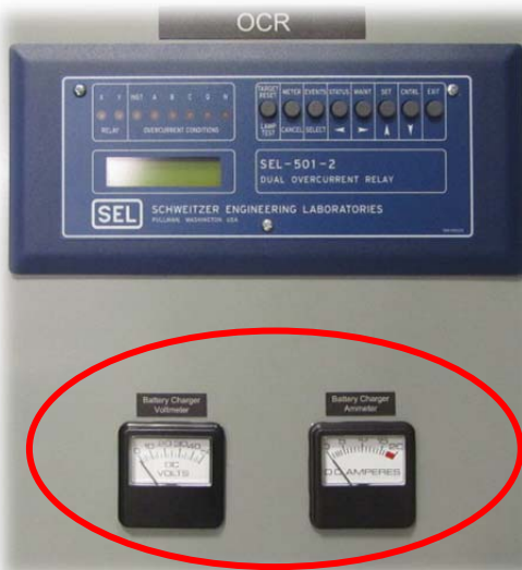
Figure 13: Self-contained Control Power Battery Charging System for Control Power
