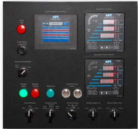
Figure 7: GP Control System Module with Integrated Lights, Sync Control Switches
