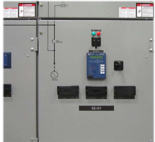
Figure 31: Generator Protection Relay Section with Mimic Bus, Pistol Grip Circuit Breaker Control Switch & Lockout Relay
