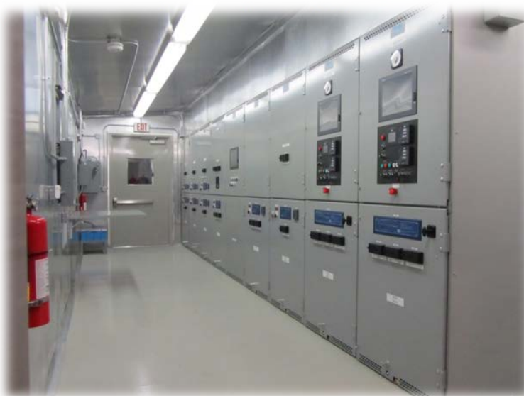
Figure 56: PwrHouse Inside Aisle of 35' Medium Voltage Utility & Generator Paralleling Switchgear E-House with Integrated Master Control
