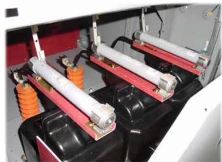
Figure 34: 5kV - Top, 15kV – Bottom Inside Open Drawer Mounted Draw-out Voltage Transformers (PTs) & Access to Primary Fuses
