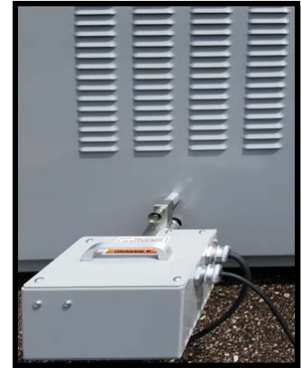
Figure 40: Electric Racking Device installed onto switchgear section circuit breaker racking mechanism
