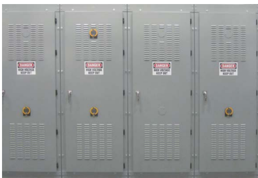
Figure 45: Rear of Non-Walk-In NEMA 3R Metal-Clad Switchgear with Hinged Rear Doors with IR Viewing Windows
