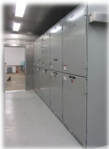
Figure 54: PwrHouse Inside Aisle of 20' Medium Voltage Metal-Clad Distribution Switchgear E-House with Isolated Operator Control Panel
