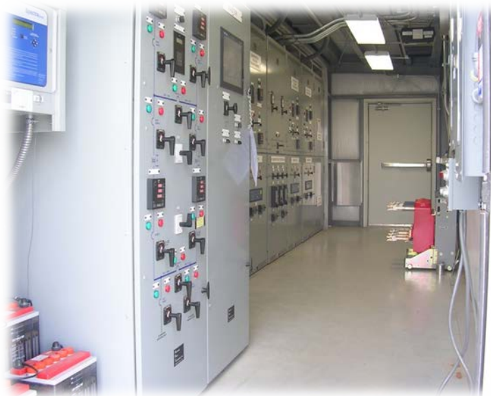
Figure 55: PwrHouse Relative Aisle Space (VCB withdrawn & in Aisleway) Includes Plenty of Space for Circuit Breaker Removal Devices
