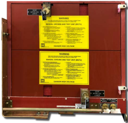
Figure 43: Manually Operated Ground & Test Device
