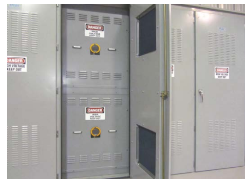
Figure 46: Rear of Walk-In NEMA 3R Metal-Clad Switchgear Enclosure with Outer Hinged Rear Doors & Inner Removeable Sheets with IR Viewing Windows
