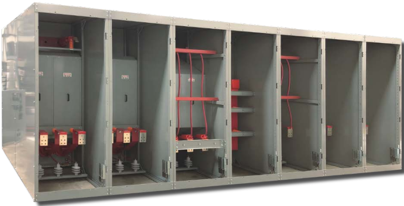
Figure 12: 15kV Max Line-Up with Rear Sheets Removed, Showing Enclosed Main Bus Compartments & Incoming/Outgoing Surge Arresters
