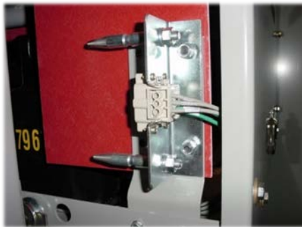
Figure 33: Auxiliary Drawer Secondary Self-Aligning Contacts
