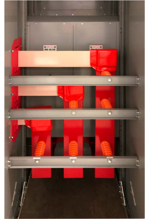
Figure 13: Inside Rear of Metal-Clad Bus Tie Section
