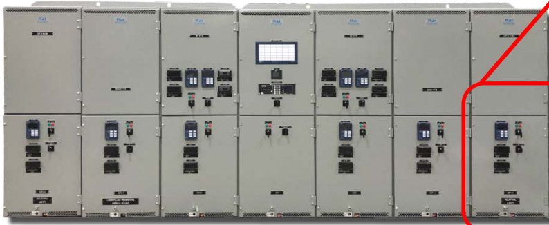
Figure 15: 15kV Main-Tie-Main Metal-Clad Switchgear Line-up
