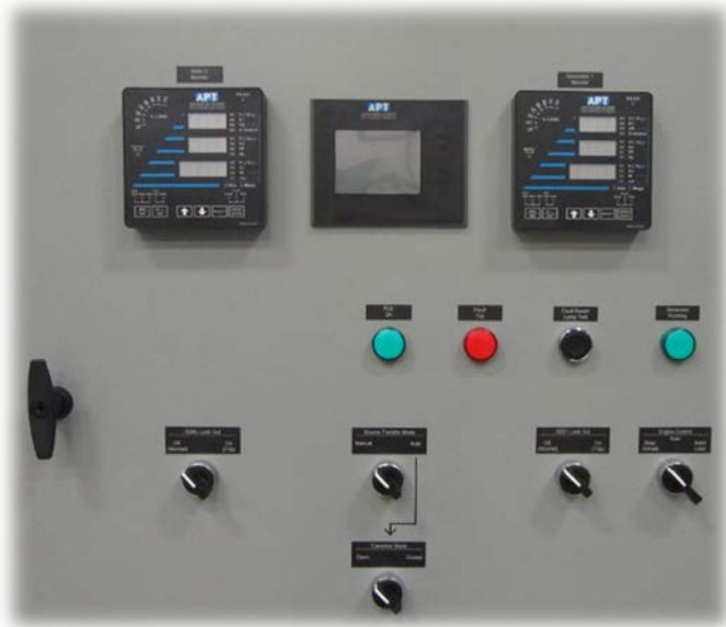
Figure 8: ATO & SL (selectable) Control System Local Operator Interface
