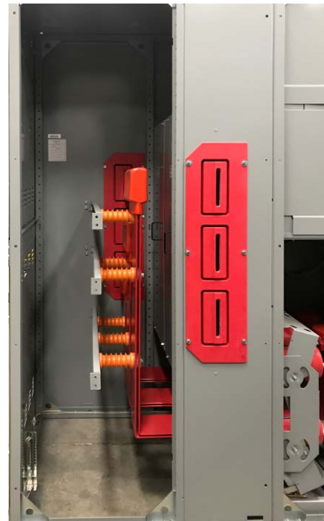
Figure 14: Side View of Bus A Connecting to Bus B in the 15kV Max Metal-Clad Bus Tie Section
