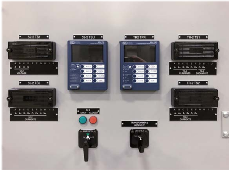
Figure 30: ANSI/IEEE 1547 Utility Intertie Protection Relays, Test Switches, Pistol Grip CB Switch & (86) Oval Handle Lockout Relay
