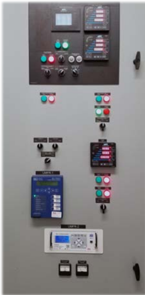
Figure 6: UP, PS, & ATC Control System Modules in Master Control Panel
