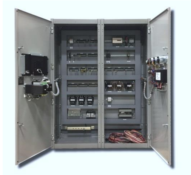
Figure 8: Generator Monitoring & Control Interior
