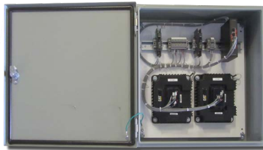
Figure 3: Two Generator Communication Conversion
