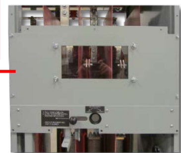
Figure 9: 15kV Max Vacuum Circuit Breaker over Vacuum Circuit*
