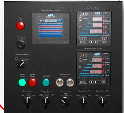
Figure 29: Close-Up of APT GP – Generator Paralleling Advanced Control Module Powered Up*
