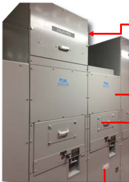
Figure 5: 5kV ATS Line-up*
