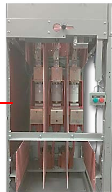
Figure 10: Close-up of Vacuum Interrupters from the front of the section*
