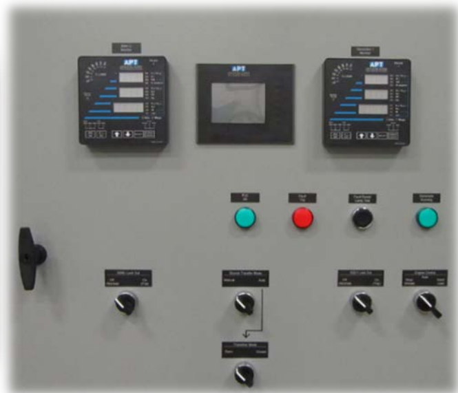
Figure 22: Control System Local Operator Interface with ATC Control Unit*
