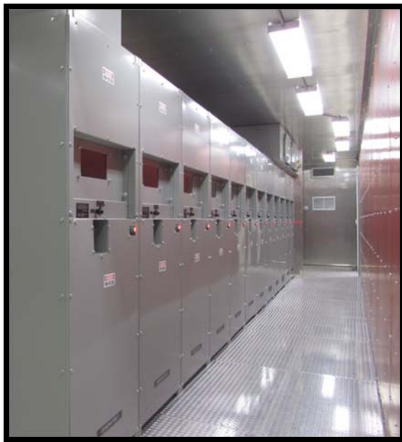
Figure 11: Inside of ISO Container based Switchgear Module with Ultra Compact Front Access (FA) Air Insulated Vacuum Circuit Breaker Switchgear
