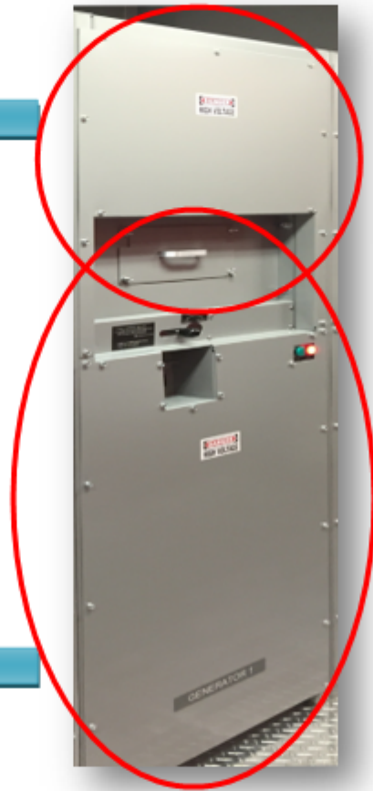
Figure 2: Single Front Access Section with Dead Fronts Attached
