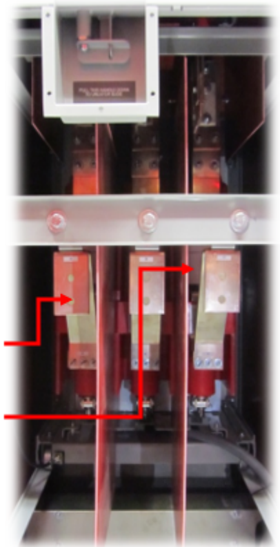
Figure 6: Inside cable connection compartment
