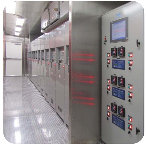
Figure 10: Front Access Switchgear, Isolated from Local and Remote Operator Control Stations gives unprecedented safety and security to Switchgear Operators in the sheltered isle
