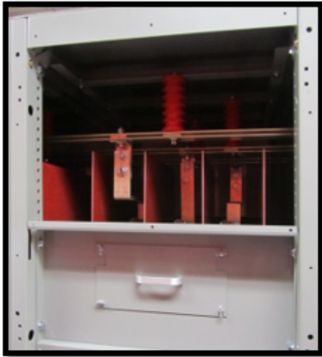
Figure 3: Dead Front Removed Exposing Main Bus Compartment with Cover Over Visual Disconnect Window
