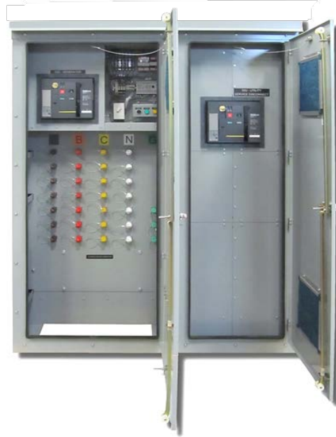
Figure 6: 2500A Service Entrance Utility & Temporary Generator Quick Connection
