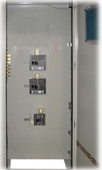
Figure 7: Auxiliary Feeder Section w/ Kirk Key Transfer Block & Interlocks
