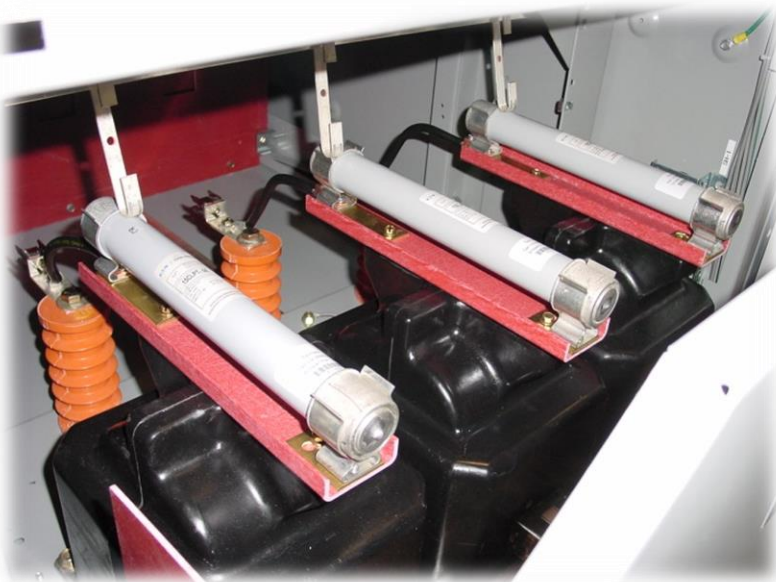
Figure 4: Carbon Steel NEMA 1 Metal Clad Type Drawout Auxiliary Drawer
