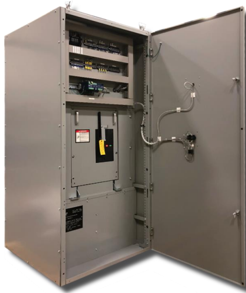
Figure 1: Metal Enclosed Generator Output Protection Switchgear
