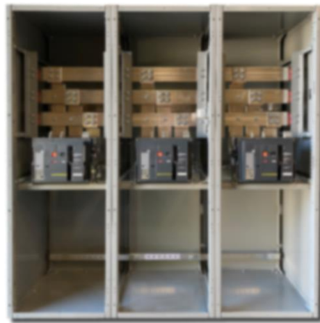
Figure 2: 500kW, 480V, 800A Paralleled Generators Disconnect & Output Protection Insulated Case Circuit Breakers and load take-off
