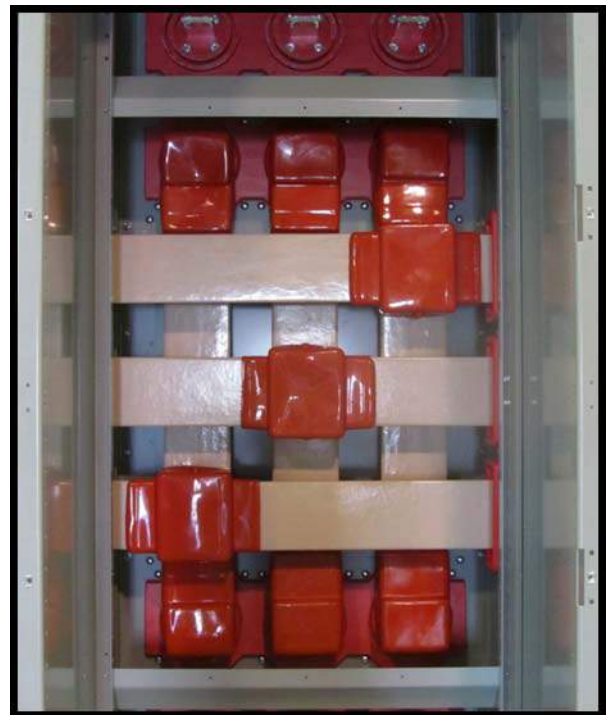
Figure 6: Close-up of insulated silver plated copper main bus
