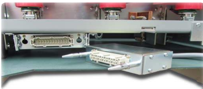
Figure 12: Test Cabinet circuit breaker connection plug to be inserted into secondary connection receptacle in rear of breaker
