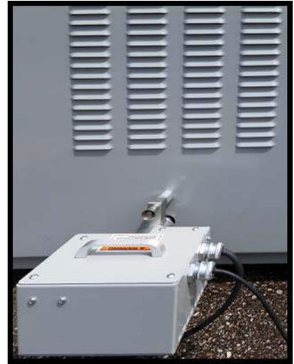
Figure 10: Electric Racking Device installed onto switchgear section circuit breaker racking mechanism
