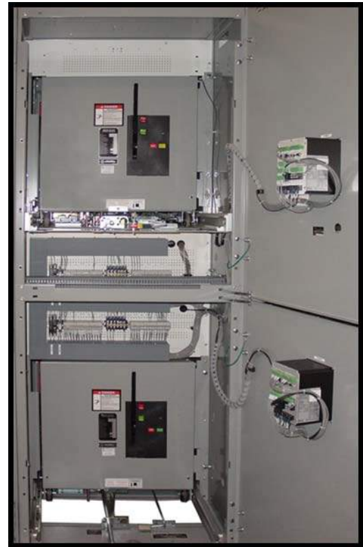
Figure 1: Breaker Over Breaker
