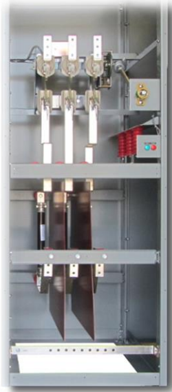
Figure 1: Indoor NEMA 1 Section Switching Device with Overcurrent Protection
