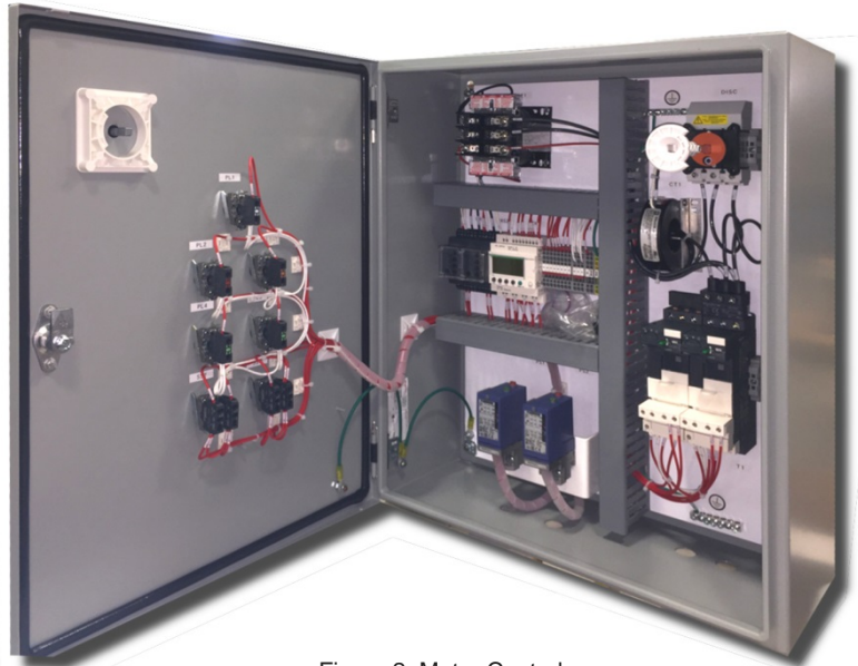
Figure 2: Motor Control & Annunciator Panel Interior NEMA 1
