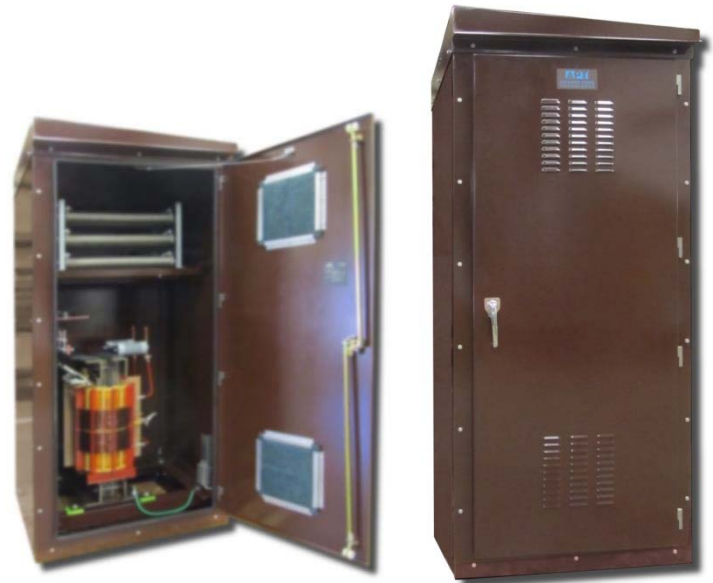
Figure 2: High Resistance Grounding System NEMA 3R Internal/External
