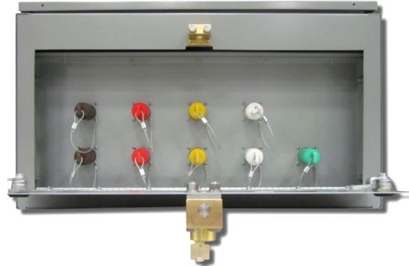
Figure 6: 800A Temporary Generator Connection Receptacles Accessed via Key
