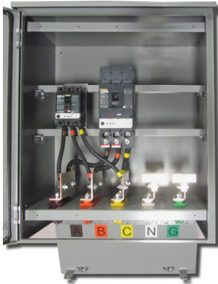
Figure 3: 600A Quick Connection with Auxiliary Circuit Breaker
