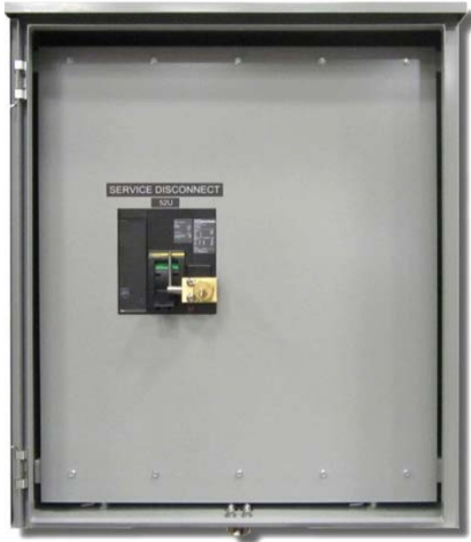
Figure 5: 800A Interlocked Utility Service Disconnect
