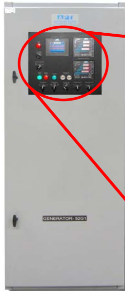
Figure 31: Generator Protection Circuit Breaker behind door & Door Mounted Generator Paralleling Control*
