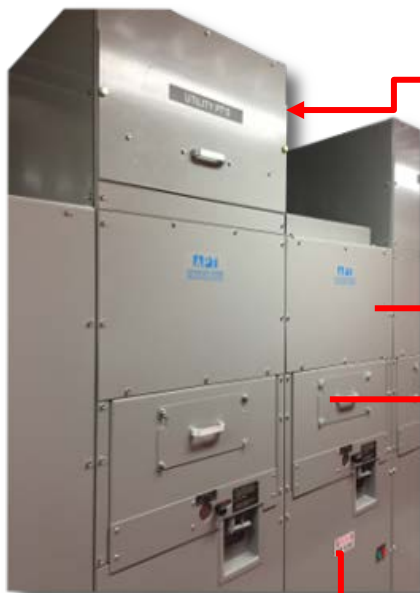
Figure 9: 5kV ATS Line-up*
