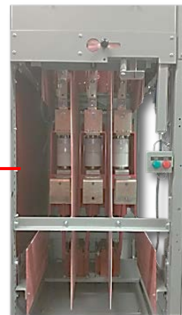
Figure 15: Close-up of Vacuum Interrupters from the front of the section*
