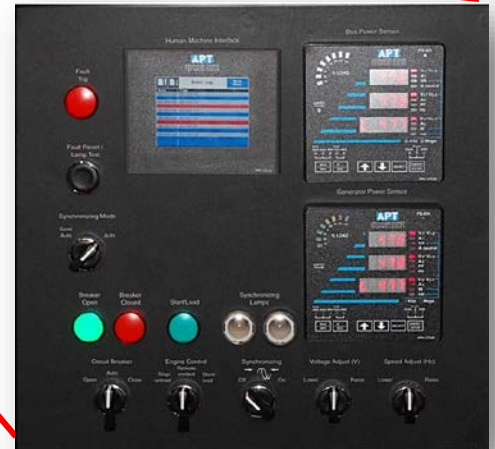
Figure 32: Close-Up of APT GP – Generator Paralleling Advanced Control Module Powered Up*
