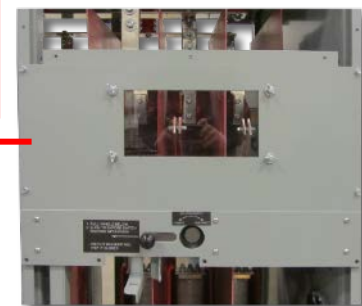
Figure 14: 15kV Max Vacuum Circuit Breaker over Vacuum Circuit*
