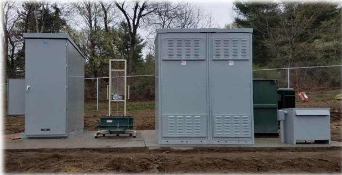
Figure 1: BrightPwr - 1MW Community Power Engineered Solar Power Collector & Protection System Pad mount NEMA 3R Non-Walk-In
