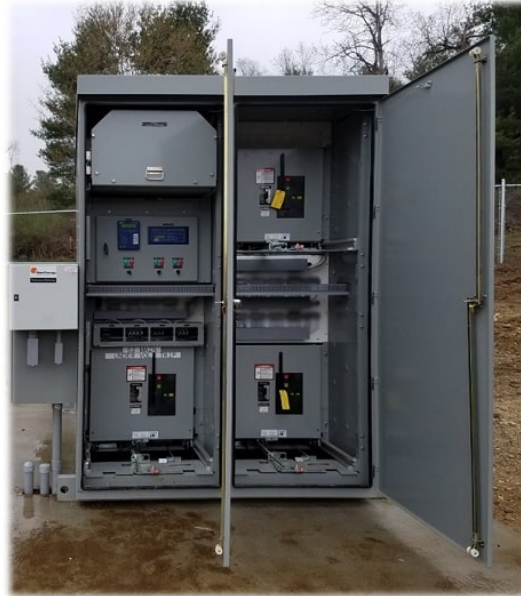
Figure 4: MEA-Series - Utility Intertie Protection & Generator Interrupter Switchgear
