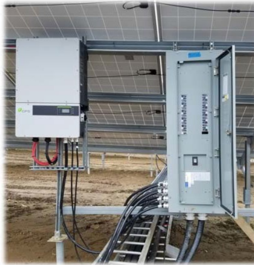
Figure 15: 600A Solar Combiner Panelboard Installed
