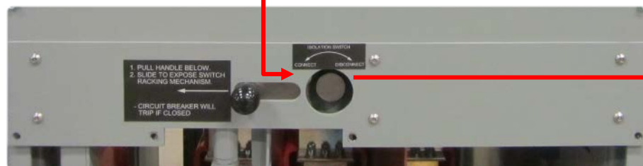
Figure 18: Access to The Racking Mechanism*
