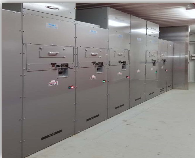
Figure 47: PwrContainer Relative Aisle Space (VCB withdrawn & in Aisleway) Includes Plenty of Space for Circuit Breaker Removal Devices*
