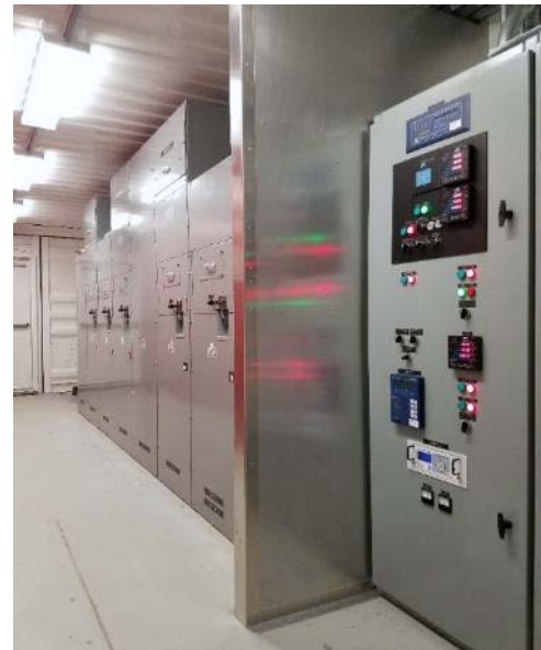
Figure 46: PwrContainer Inside Aisle of 30' Medium Voltage Utility & Generator Paralleling & Automatic Transfer Switchgear E-House with Isolated Master Control Panel*
