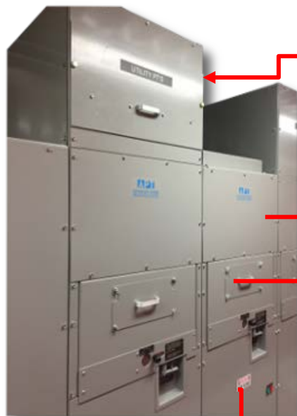
Figure 4: 5kV ATS Line-up*
