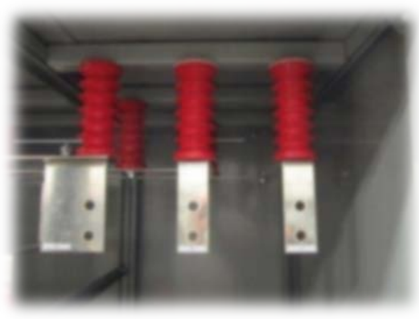
Figure 23: Load Take-Off Connection*
