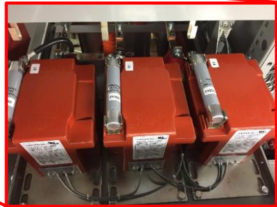
Figure 38: 5kV - Top, 15kV - Bottom Drawer Mounted Voltage Transformers (PTs) & Access to Primary Fuses*
