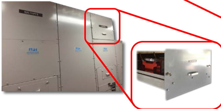
Figure 39: Auxiliary Drawer with Self-Aligning Contacts*
