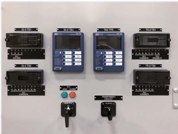
Figure 35: ANSI/IEEE 1547 Utility Intertie Protection Relays, Test Switches, Pistol Grip CB Switch & (86) Knob Grip Lockout Relay*
