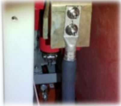
Figure 21: Power Source Cable Connection*
