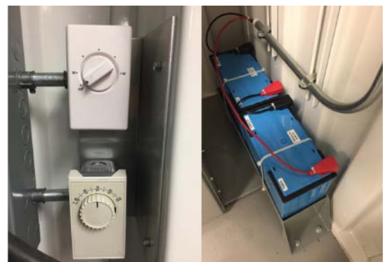
Figure 48: PwrContainer Inside Temperature Controls with 24VDC Battery Rack* *
