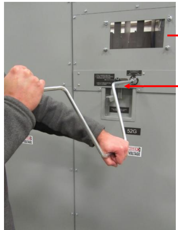
Figure 19: Operation of Isolation Switch to Create Visible Disconnect *
