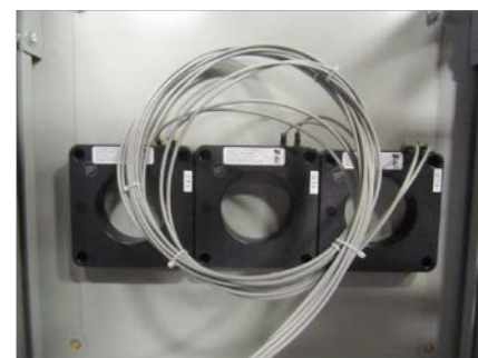
Figure 41: Relaying and metering Current Transformers (CTs)*
