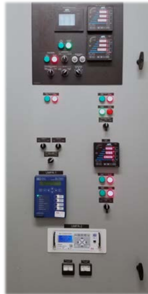
Figure 13: ATC, SL1, IM, IE Control System Modules in Master Control Panel*
