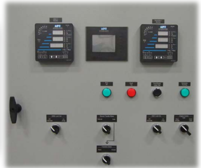
Figure 15: Control System Local Operator Interface with Premium Control Unit*
