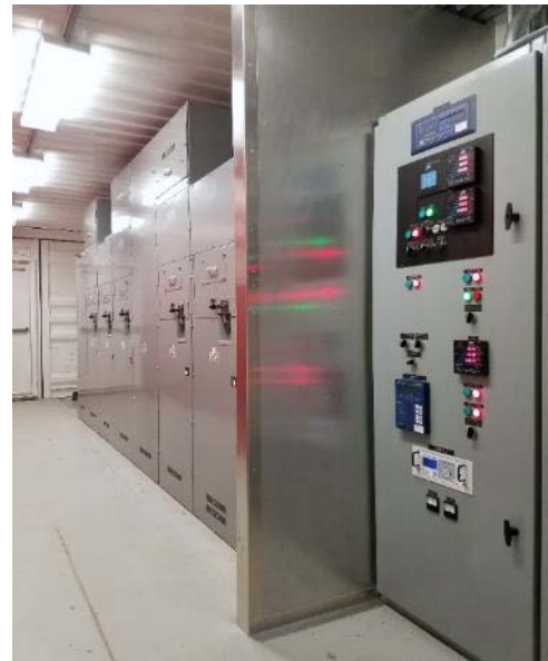
Figure 50: PwrContainer Inside Aisle of 30' Medium Voltage Utility & Generator Paralleling & Automatic Transfer Switchgear E-House with Isolated Master Control Panel*
