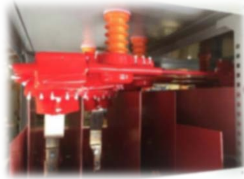
Figure 26: Optional Insulated Main Bus*
