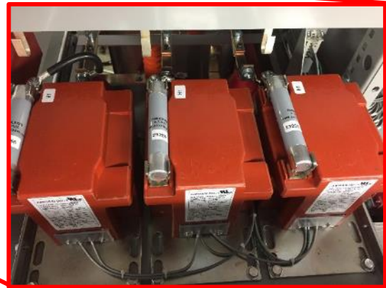
Figure 43: 5kV - Top, 15kV - Bottom Drawer Mounted Voltage Transformers (PTs) & Access to Primary Fuses*
