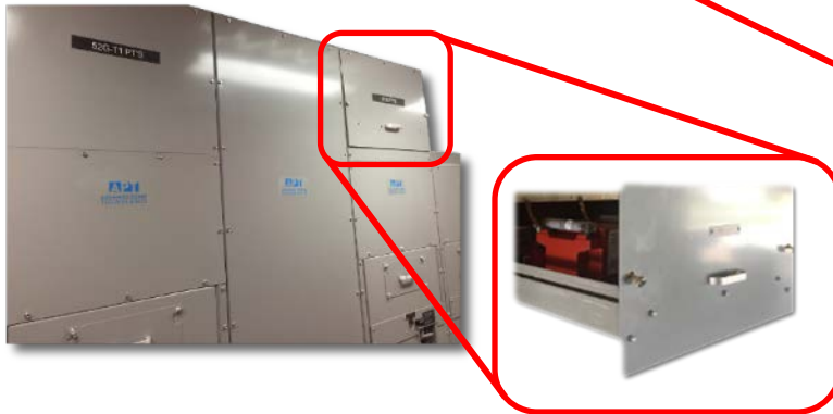
Figure 42: Auxiliary Drawer with Self-Aligning Contacts*
