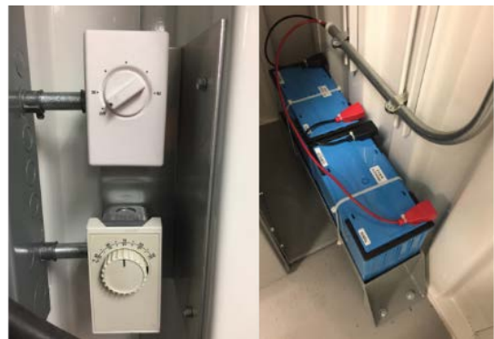
Figure 52: PwrContainer Inside Temperature Controls with 24VDC Battery Rack* *
