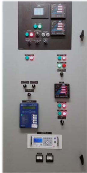
Figure 16: ATC, SL, IM, IE Control System Modules in Master Control Panel*
