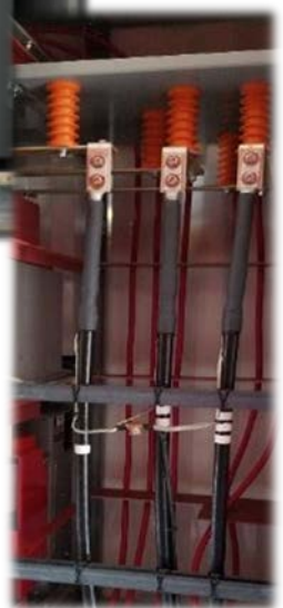
Figure 29: Load Take-Off Cable Connections*
