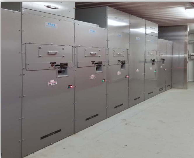
Figure 51: PwrContainer Relative Aisle Space (VCB withdrawn & in Aisleway) Includes Plenty of Space for Circuit Breaker Removal Devices*
