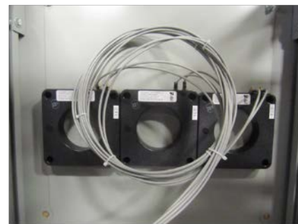
Figure 45: Relaying and metering Current Transformers (CTs)*
