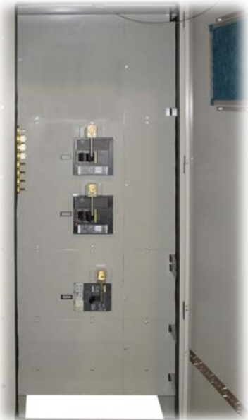
Figure 7: Auxiliary Feeder Section w/ Captive Key Transfer Block & Interlocks
