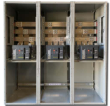
Figure 6: 500kW, 480V, 800A Paralleled Generators Disconnect & Output Protection Insulated Case Circuit Breakers and load take-off
