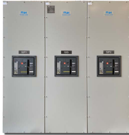
Figure 5: Three (3) 750kW, 480V, 1200A Paralleled Generator Disconnect & Output Protection Insulated Case Circuit Breaker Lineup with Front Removable Sheets
