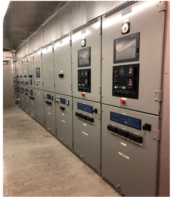
Figure 29: MEA Series Switchgear with Integrated Master Controls integrated into a PwrHouse Walk-In Equipment Enclosure
