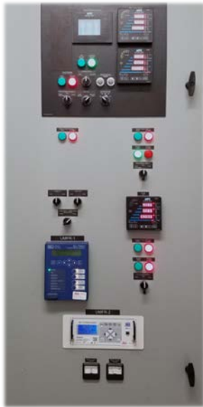
Figure 32: UP, PS, & ATC Control System Modules in Master Control Panel
