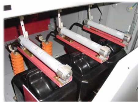
Figures 23 (top) & 24 (bottom): 5kV - Top, 15kV - Bottom Inside Open Drawer Mounted Draw-out Voltage Transformers (PTs) & Access to Primary Fuses
