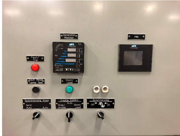
Figure 1: Switchgear Control Panel View of Typical Section*
