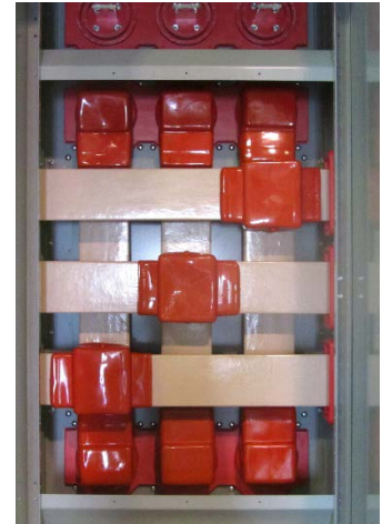
Figure 39: Interior View of Insulated Main Bus
