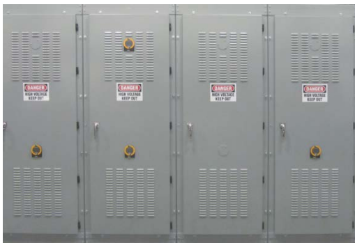
Figure 47: Rear of Non-Walk-In NEMA 3R Metal-Clad Switchgear with Hinged Rear Doors with IR Viewing Windows
