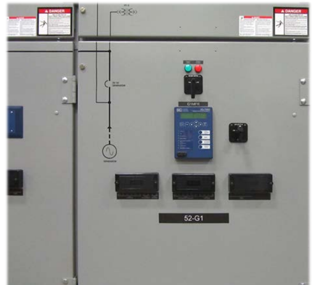
Figure 27: Generator Protection Relay Section with Mimic Bus, Pistol Grip Circuit Breaker Control Switch & Lockout Relay
