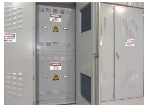
Figure 48: Rear of Walk-In NEMA 3R Metal-Clad Switchgear Enclosure with Outer Hinged Rear Doors & Inner Removeable Sheets with IR Viewing Windows
