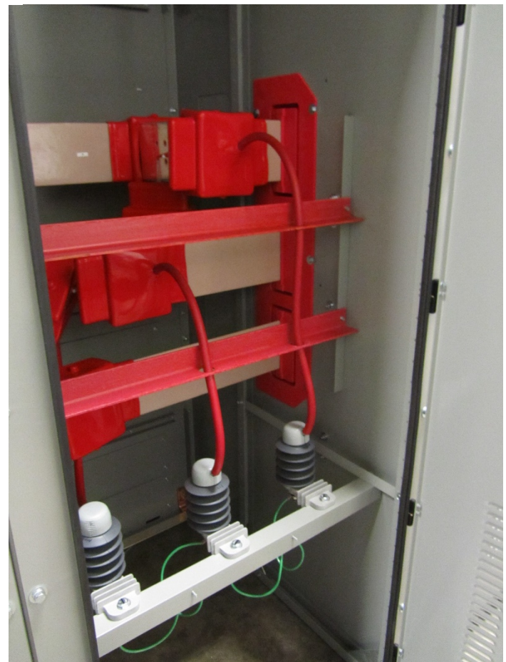
Figure 40: Side View of MEA Series Insulated Main Bus
