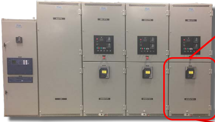
Figure 4: 15kV Metal Enclosed Vacuum Circuit Breaker Switchgear Line-up
