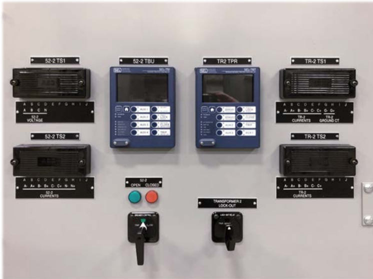
Figure 26: ANSI/IEEE 1547 Utility Intertie Protection Relays, Test Switches, Pistol Grip CB Switch & (86) Oval Handle Lockout Relay
