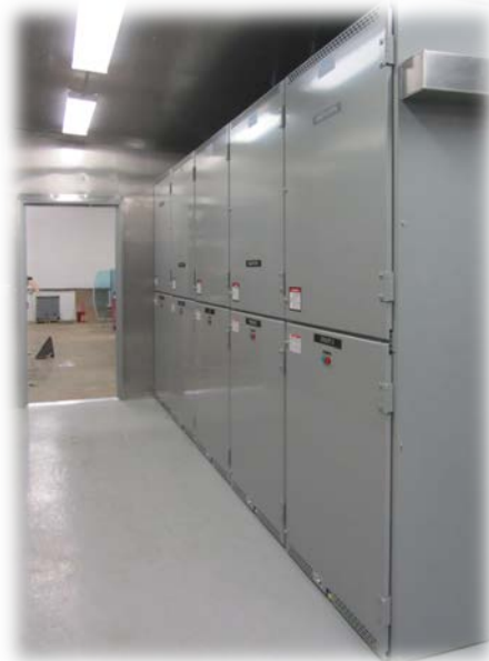
Figure 53: PwrHouse Inside Aisle of 20' Medium Voltage Metal-Clad Distribution Switchgear E-House with Isolated Operator Control Panel
