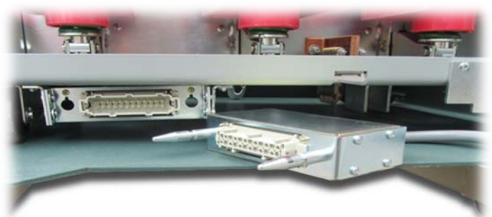
Figure 44: Test Cabinet circuit breaker connection plug to be inserted into secondary connection receptacle in rear of breaker
