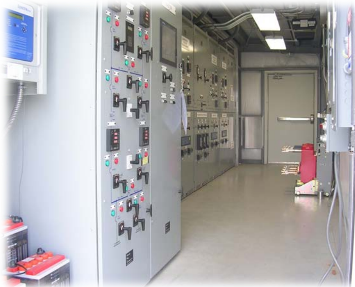
Figure 54: PwrHouse Relative Aisle Space (VCB withdrawn & in Aisleway) Includes Plenty of Space for Circuit Breaker Removal Devices
