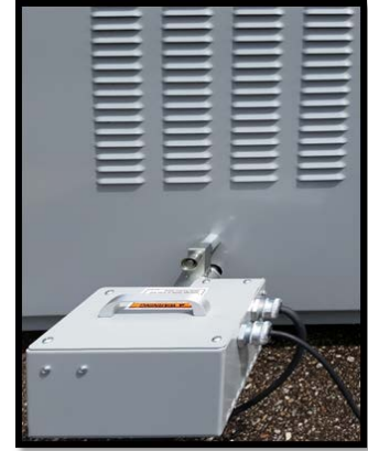
Figure 42: Electric Racking Device installed onto switchgear section circuit breaker racking mechanism
