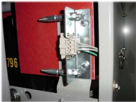
Figure 22: Auxiliary Drawer Secondary Self-Aligning Contacts
