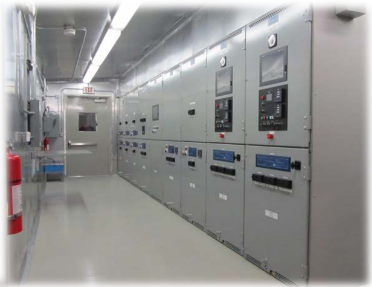
Figure 55: PwrHouse Inside Aisle of 35' Medium Voltage Utility & Generator Paralleling Switchgear E-House with Integrated Master Control
