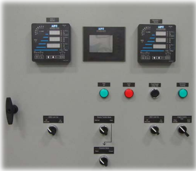
Figure 34: ATO & SL (selectable) Control System Local Operator Interface
