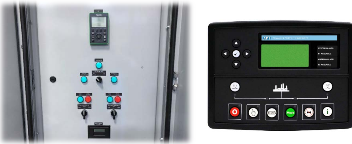
Figure 5: Standard ATS System Controllers consisting of ATO - Automatic Standby Open Transition Transfer with NA - Non-Automatic Operator Supervised Return to Normal Control
