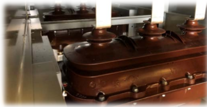
Figure 3: Sealed SF6 Gas Insulated Switching Device
