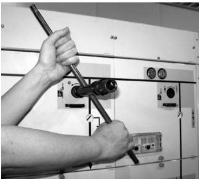
Switch disconnector
