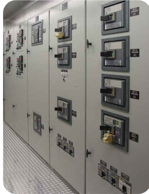
Figure 2: Interior of Low Voltage 40' Mobile PwrContainer-Based Walk-in SBU Switchgear
