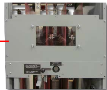
Figure 12: 15kV Max Vacuum Circuit Breaker over Vacuum Circuit*
