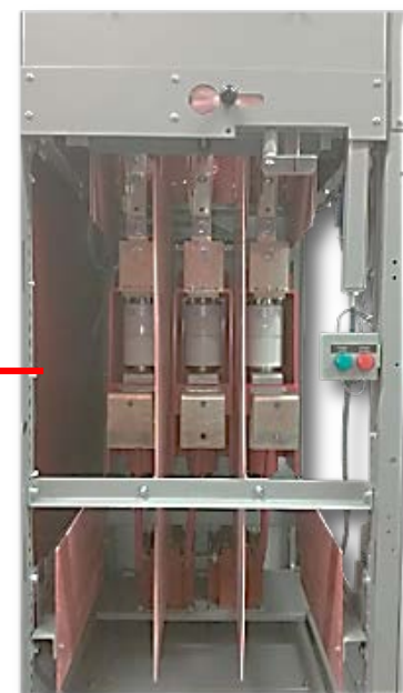
Figure 12: 15kV Max Vacuum Circuit Breaker over Vacuum Circuit*
