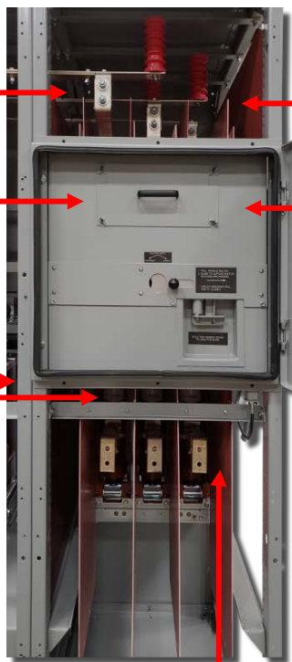
Figure 14: 5kV ATS Typical Generator Section Configuration*
