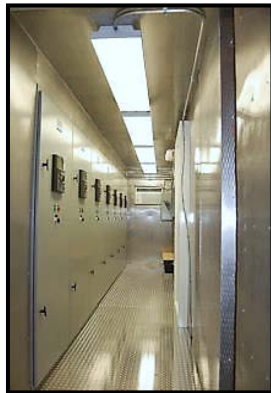
Figure 4: 20' Inside ISO Container-Based Walk-in Switchgear Module
