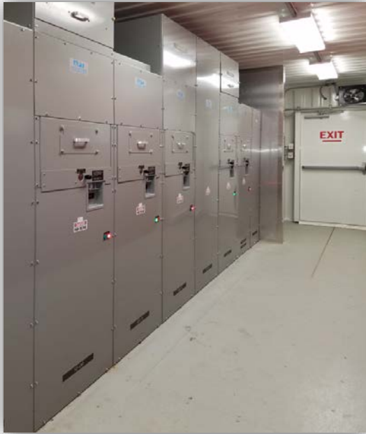
Figure 1: Interior of Medium Voltage 40' Mobile PwrContainer-Based Walk-in FAC Switchgear
