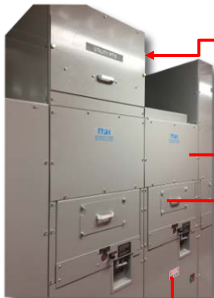
Figure 9: 5kV ATS Line-up*
