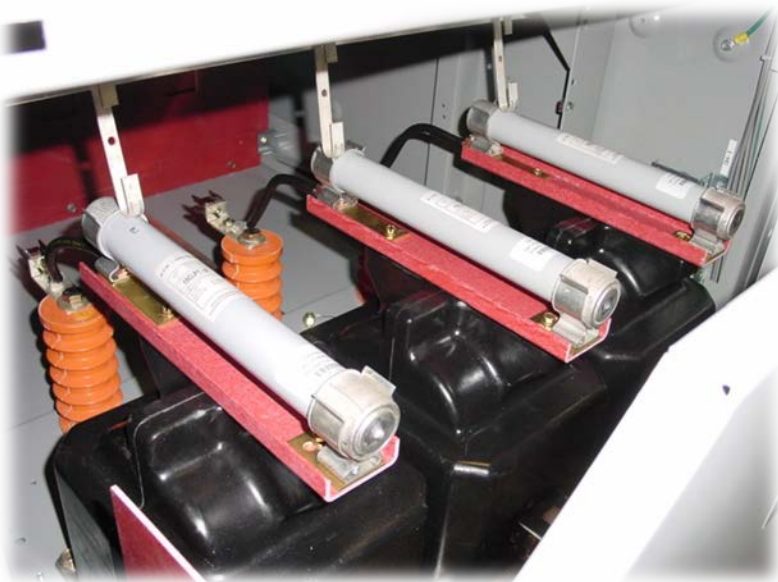
Figure 17: Carbon Steel NEMA 1 Metal Clad Type 15kV Drawout Auxiliary Drawer
