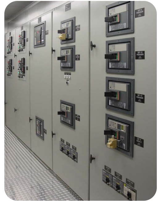
Figure 4: Low voltage Switchgear inside Container Module
