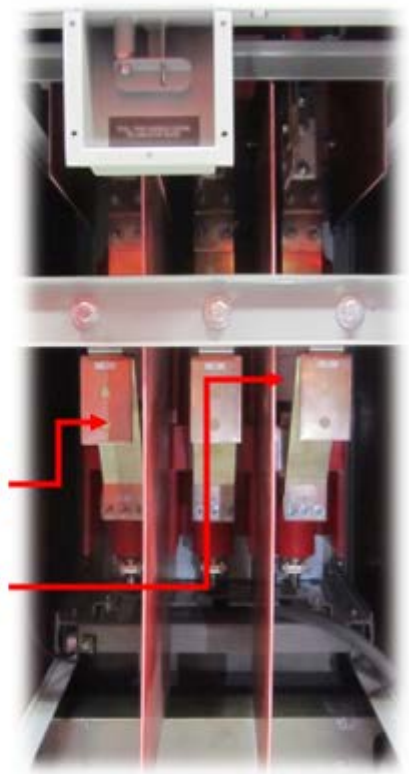
Figure 6: Inside cable connection compartment
