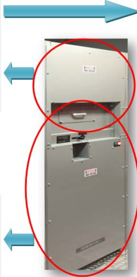
Figure 2: Single Front Access Section with Dead Fronts Attached
