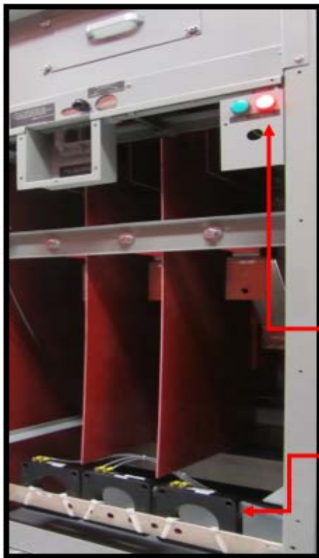
Figure 5: Cable Connection Compartment Dead Front Removed
