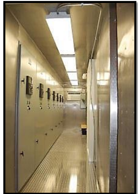
Figure 6: 20' Inside ISO Container-Based Walk-in Switchgear Module
