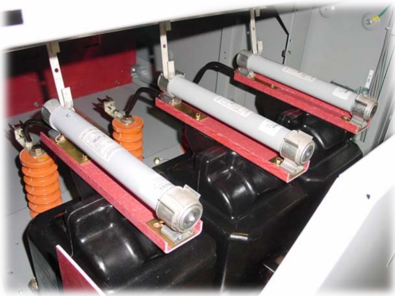
Figure 4: Carbon Steel NEMA 1 Metal Clad Type 15kV Drawout Auxiliary Drawer
