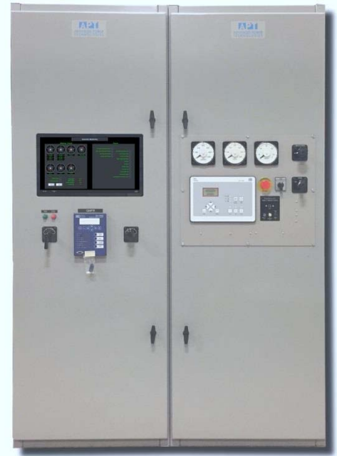
Figure 9: Generator Monitoring & Control Panel with Analog & Digital Metering & Relays
