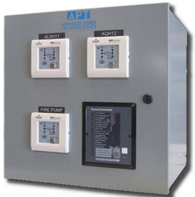
Figure 12: APT Emergency Power Monitoring Panel for Three Automatic Transfer Switches & One Cummins Generator
