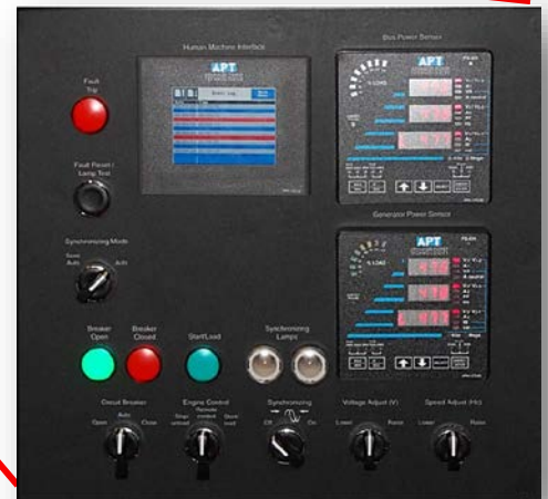
Figure 5: Close-Up of APT GP Advanced Control Module Powered Up
