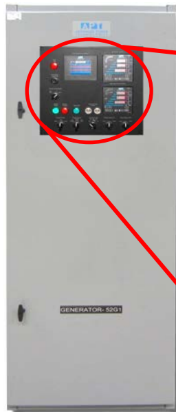
Figure 4: Generator Protection Circuit Breaker behind door & Door Mounted Generator Paralleling Control
